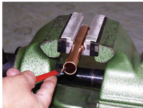
2. Deburring of the pipe extremities inside and outside
