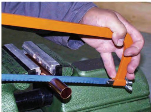
1. Rectangularly saw off the pipes
