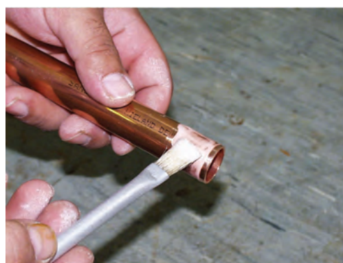
4. Apply the soldering flux on the pipe
