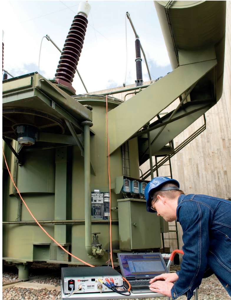
IDAX 300 (here controlled by an external PC) is a powerful tool for condition assessments of power transformers.
