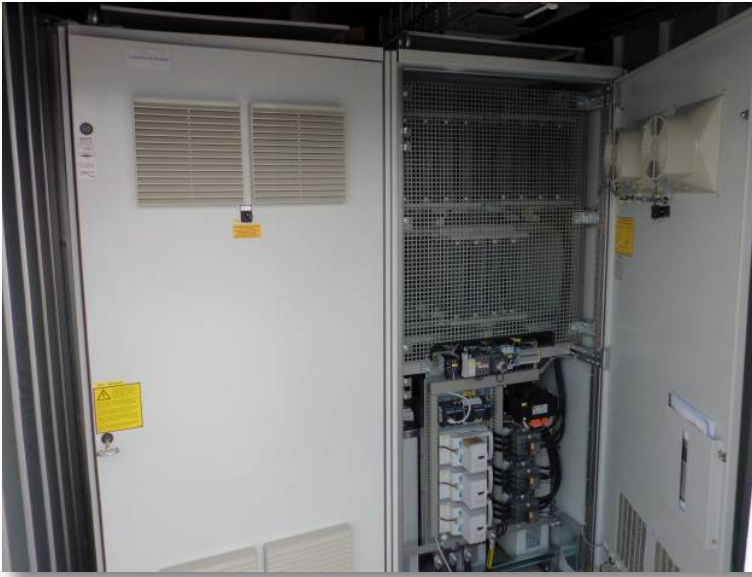
Figure 8: Passive Harmonic Filter from Condensator Dornit
