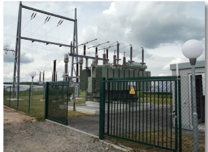
Figure 3: Tauberland Solar Park – 110/20-kV Transformer
