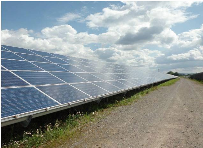
Figure 2: Tauberland Solar Park – Photovoltaic Panels
