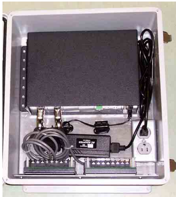
Figure 37 Contained in NEMA Enclosure – 61STD unit connected to voltage and current input pods; power source assembly is shown on the right.
