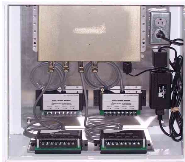
Figure 34 Contained in NEMA 4 Pod Enclosure – 61STD unit connected to two each of voltage and current input pods; power source assembly is shown on the right in a NEMA 4 Data Enclosure.
