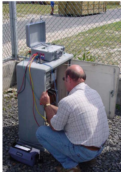
Fig. 1: An on-site test with METES 320
