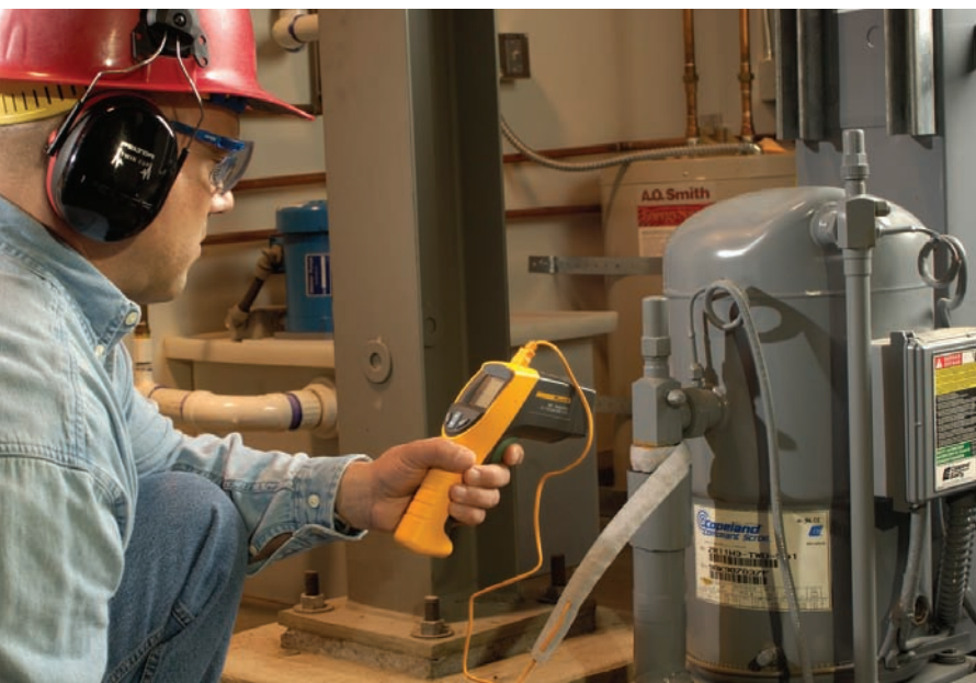
Taking a contact temperature measurement at the compressor outlet on the liquid line.
